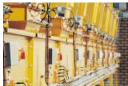
One AS-i flat cable instead of many parallel cables: In a brewery the interface serves to transfer the sensor signals to the higher-level controller.
