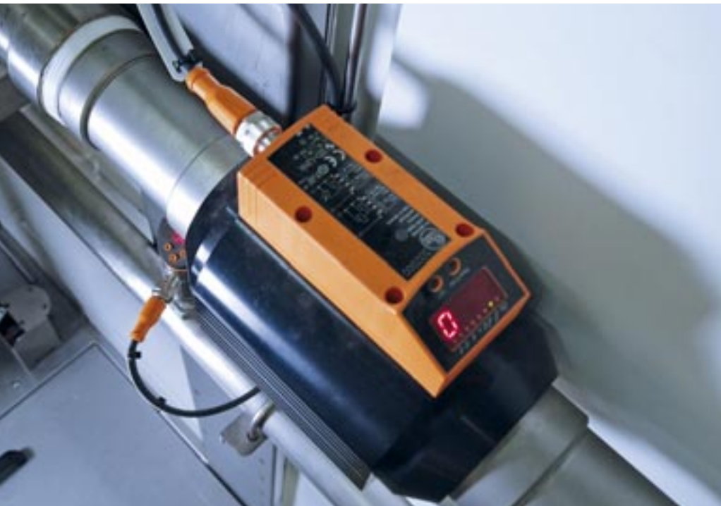
The airflow used for drying is measured using the SD2000.
