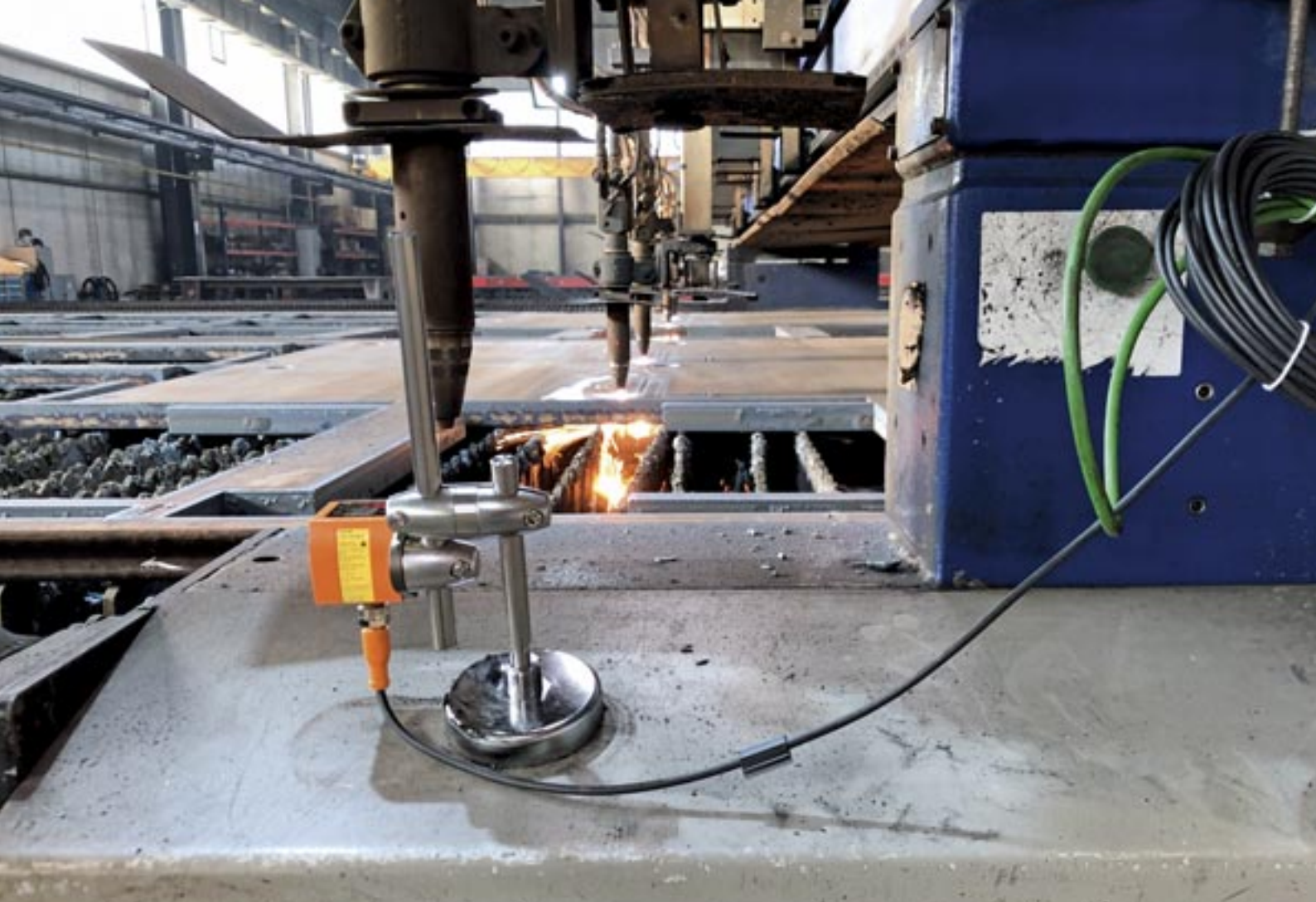
The distance sensor O1D108 detects whether the cutting head is in operation or in the rest position by means of time-of-flight measurement.
