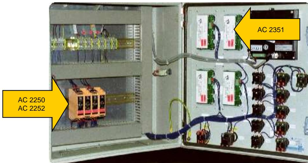
**Figure 3: Combination of an illuminated push-button module for front panel mounting (AC2351) and SmartLine control cabinet modules (AC2250, AC2251)**
