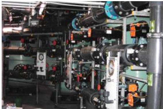
**Figure 5: quarter-turn actuators with AS-i: Address, connect, ready!**
