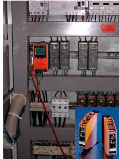
**Photo 10: AS-i ControllerE for valve controlling filter circuits 1+2
