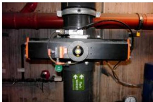
**Figure 6: premounted quarter-turn actuator of the IND/T5 series.**
