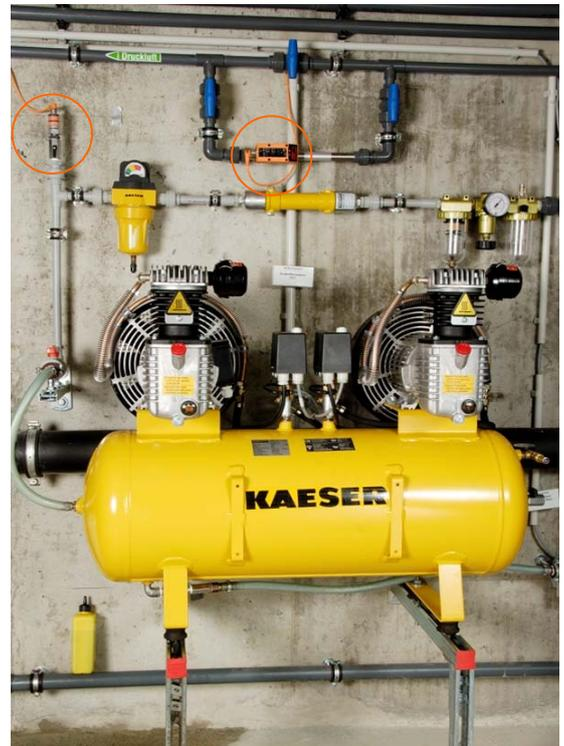
Figure 10: Compressed air generation via dual compressor with pressure sensor PK6524 and compressed air meter SD6000.
