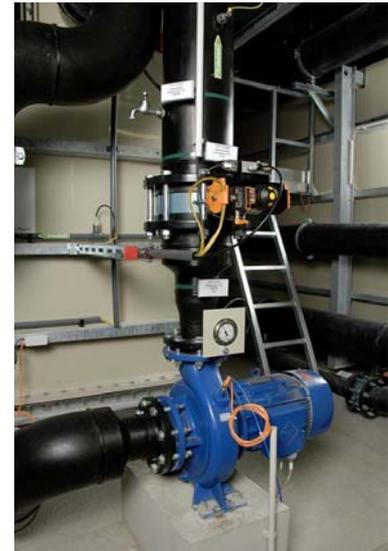
Figure 14: Filtrate pumps at the filters
