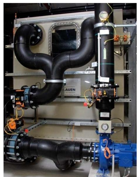
Figure 6: Filter by WTA with AS-i modules AC2516 and AC2507
