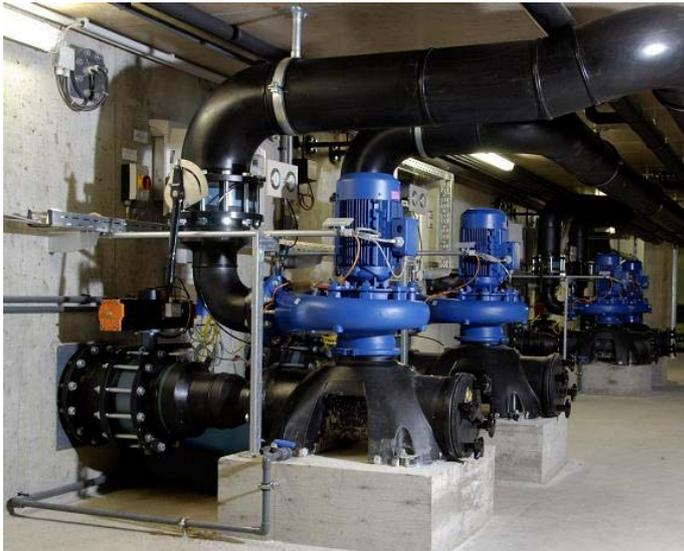
Figure 13: 4 raw water pumps at the splash containers
