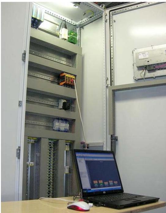
Figure 15: Use of the VSE002 diagnostic electronics, on-site diagnosis via laptop
