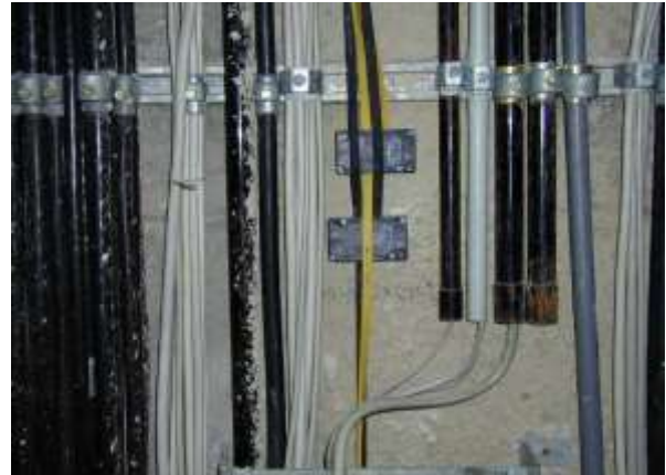
Figure 5: Comparison of conventional wiring and AS-Interface with the example of a flat cable branching
