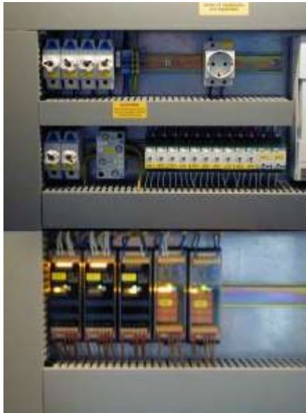
Figure 3: Data transfer via relay contact (4I/4O modules)
