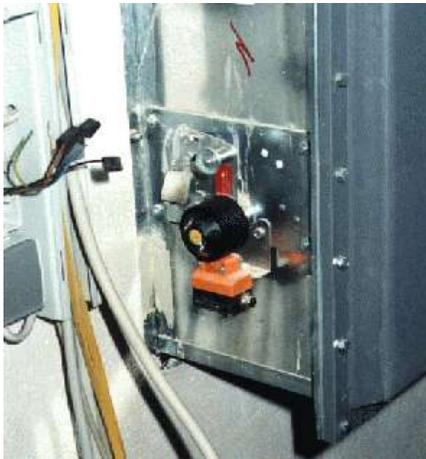
**Ind. dual sensor IND T5 with corresponding puck. AS-i interface directly integrated in the sensor.**
