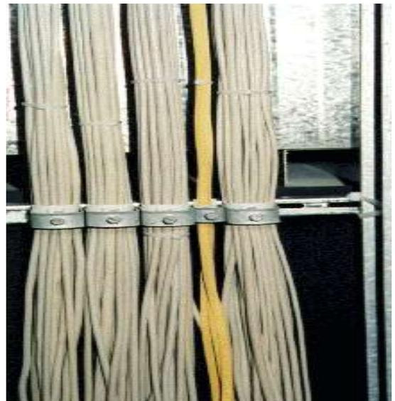
Common parallel wiring to the control cabinet requires high mounting efforts. AS-i transfers data and ensures the voltage supply of the sensors via one two-wire cable.
