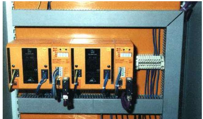
In the control cabinet no more I/O modules are required. AS-i transfers data and ensures the voltage supply of all sensors in the field.
