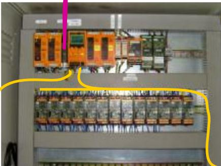
Figure 6: interior view control cabinet 1 (microfiltration 1 + control bioreactors)
