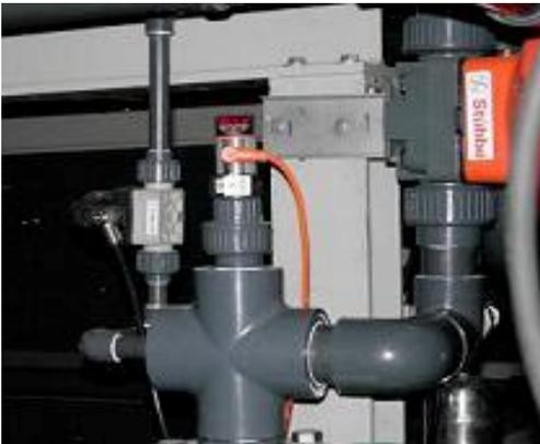
**Figure 19: Pressure sensor of the PF series for system pressure measurement downstream of the booster pump controlled by a frequency converter**
