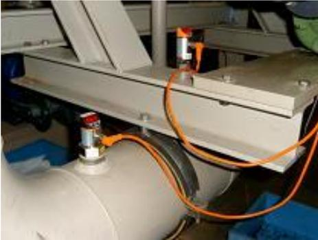
**Figure 21: Use of PF pressure sensor and TR temperature control monitor in the pressure pipe**
