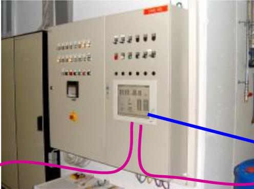
Figure 4: control cabinet 1 + control cabinet 2 with integrated industrial PC as central visualisation and controller
