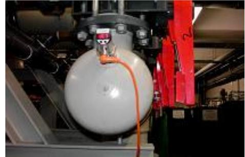
**Figure 18: Pressure sensor of the PF series with flush diaphragm for pressure measurement in microfiltration**
