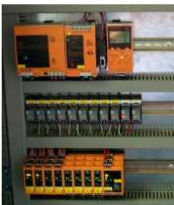
**Figure 12: AS-i SmartLine control cabinet modules (lower row)**
