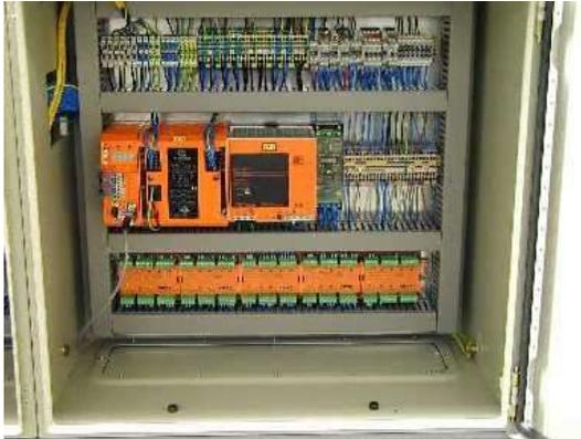
As can be seen in photo 7, the installation in the control cabinet has been reduced to a minimum. Only 5 AS-i control cabinet modules (4DI/4DO on the lowest DIN rail) for binary signals and a PT100 input module (4 inputs, next to the 24VDC power supply) for temperature measurement are located in the control cabinet next to the controller (ifm type AC1024, with 2 RS232C interfaces). All further inputs and outputs are detected via AS-i I/O modules and AS-i system solutions in the field.
