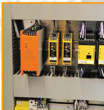
The central control components of the AS-i network
