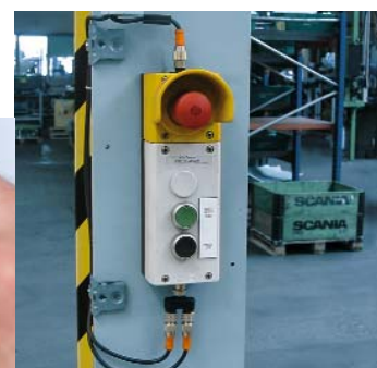
Operating element with AS-i compatibility in the automotive industry.
