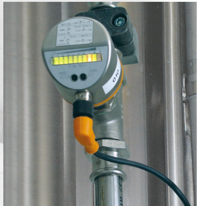
Type SI flow sensor in a cooling water monitoring application.
