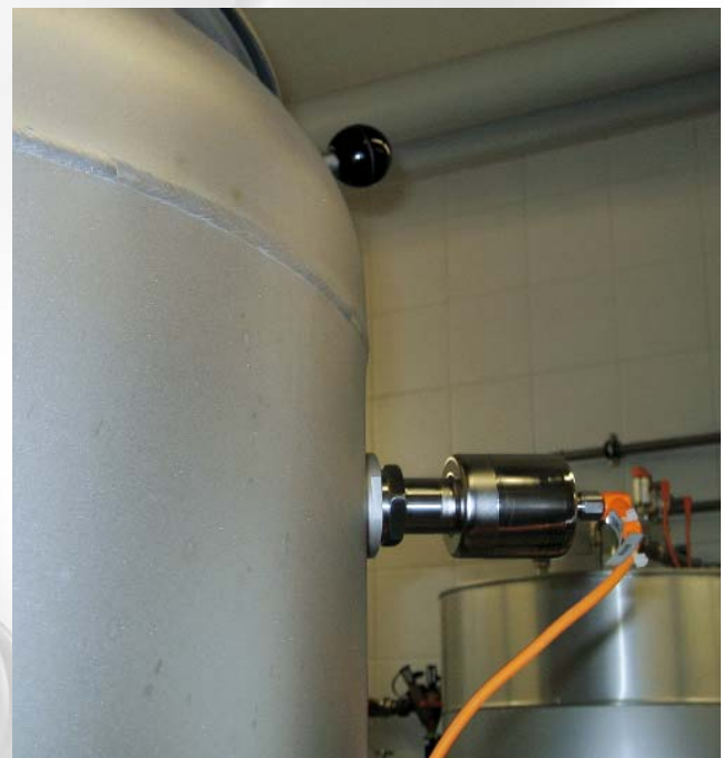
TAD temperature transmitters in hygienic applications for CIP and SIP
